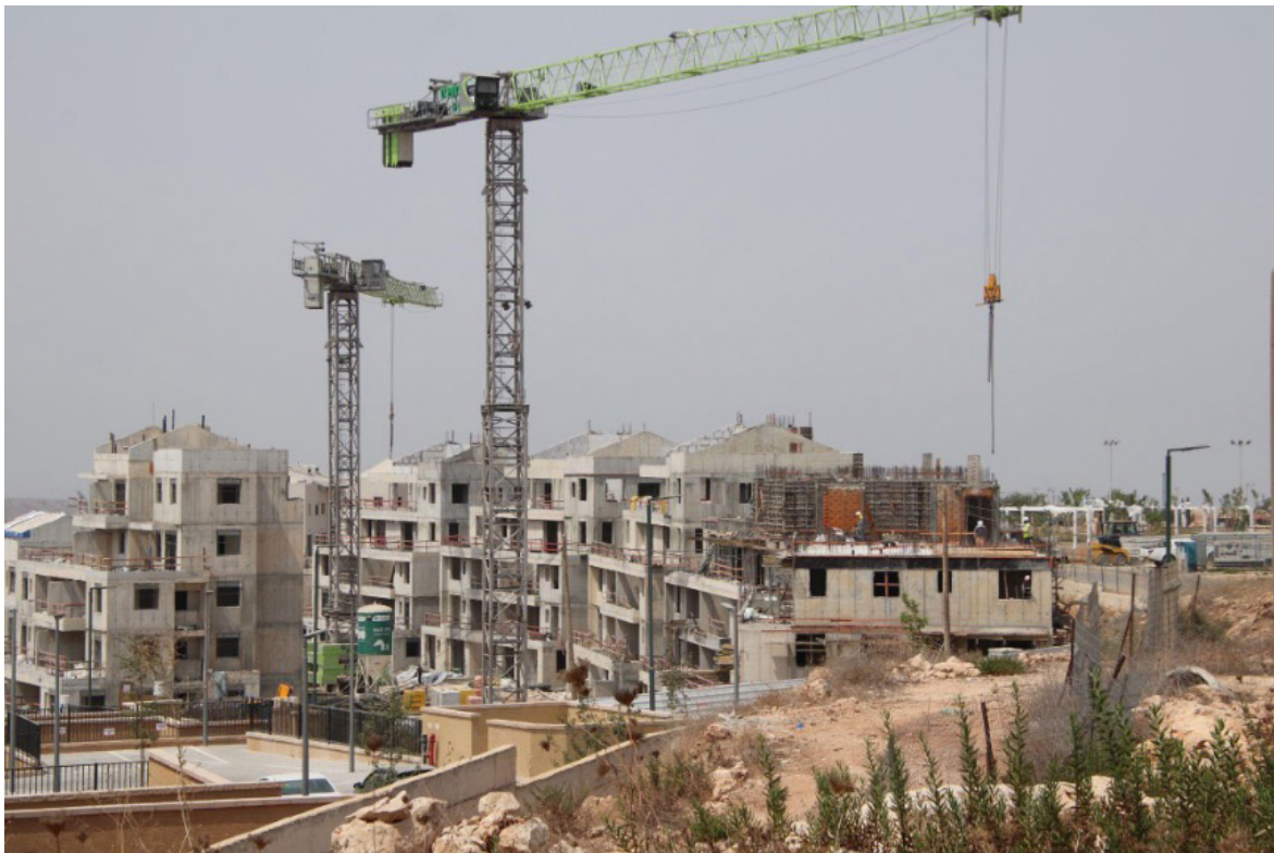
Construction site in Ofarim settlement.
