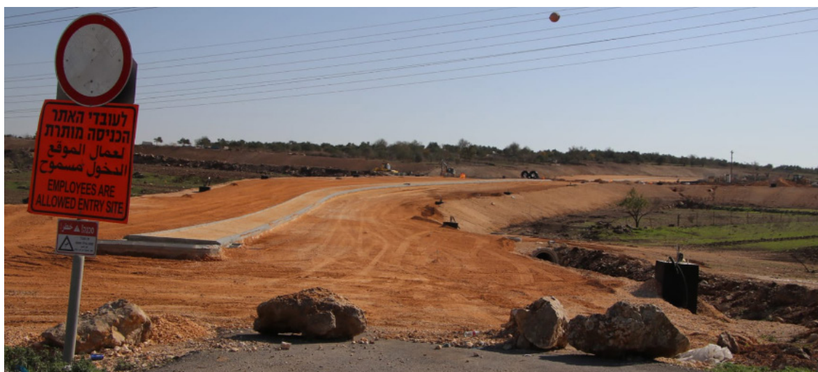
Construction work on the al-Funduq bypass road.
