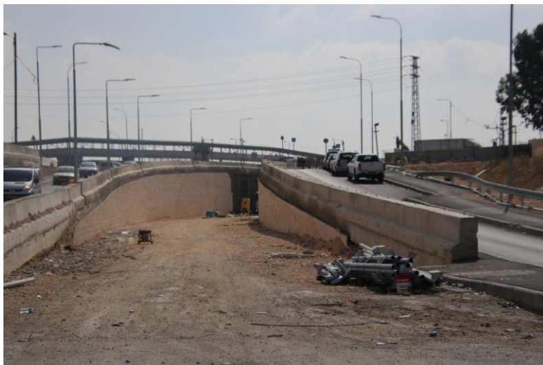
The Qalandiya Underpass
