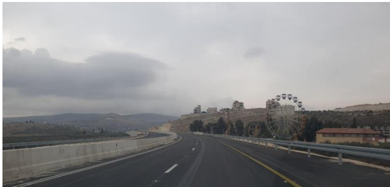
The Huwara Bypass Road
