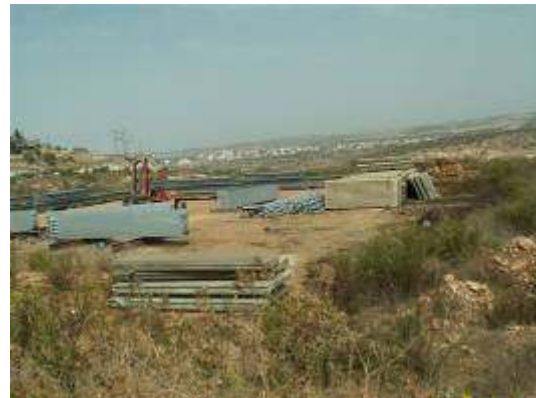
Workshop for Caravans' Construction in Elkana
